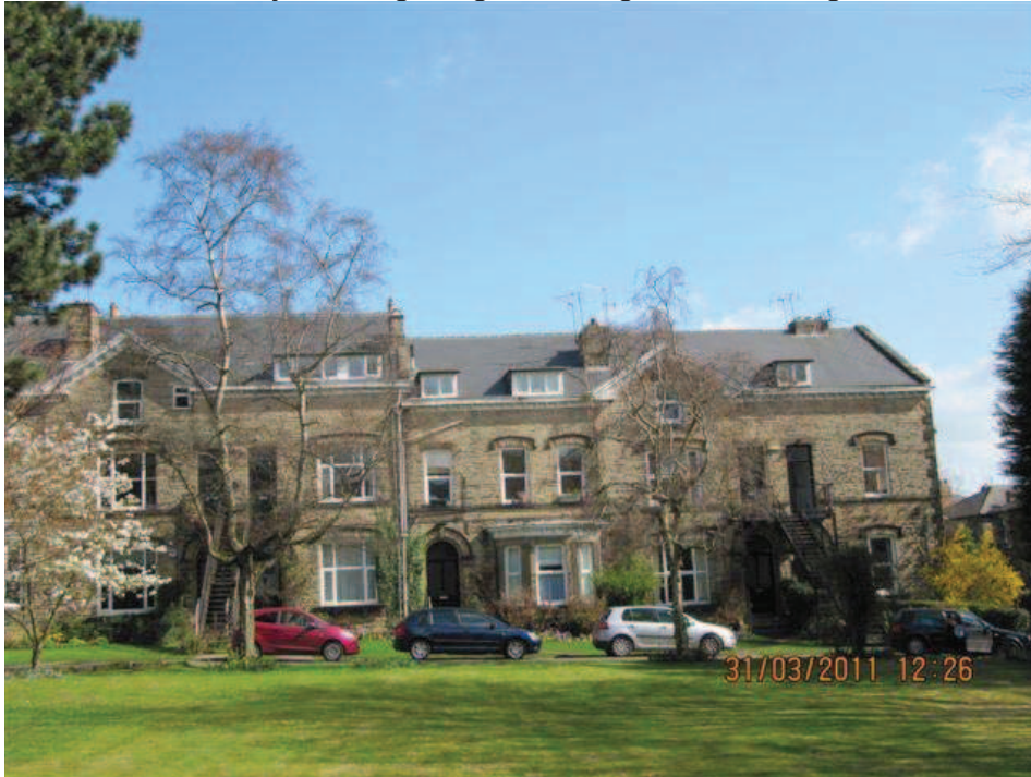
Photo of Previously Existing Bargeboarding and Guttering
